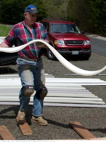
**USE GLOVES FOR SAFE HANDLING** With the board's temperature now at 220°F or higher, the probe is extracted and the insulation and top blanket removed. The decking—now the consistency of a big, hot noodle—is quickly carried to the bending jig.
